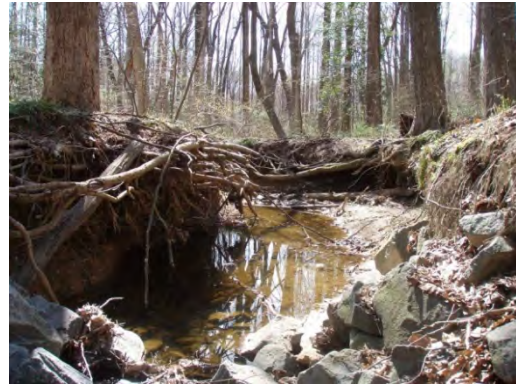
Before stream restoration-Snakeden Branch at Reach 15. Photo courtesy Nicki Bellezza.
